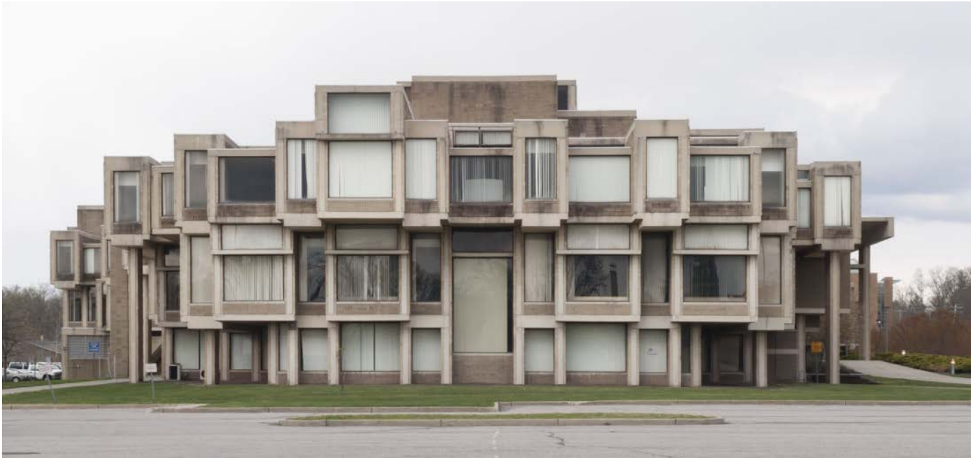
Southwest Elevation, Orange County Government Center, 2012, Goshen, NY. Photo by Sean Hemmerle. From the 2013 Graham Foundation Individual Grant to Sean Hemmerle and William Watson for Brutal Legacy: Paul Rudolph's Orange County Government Center.
